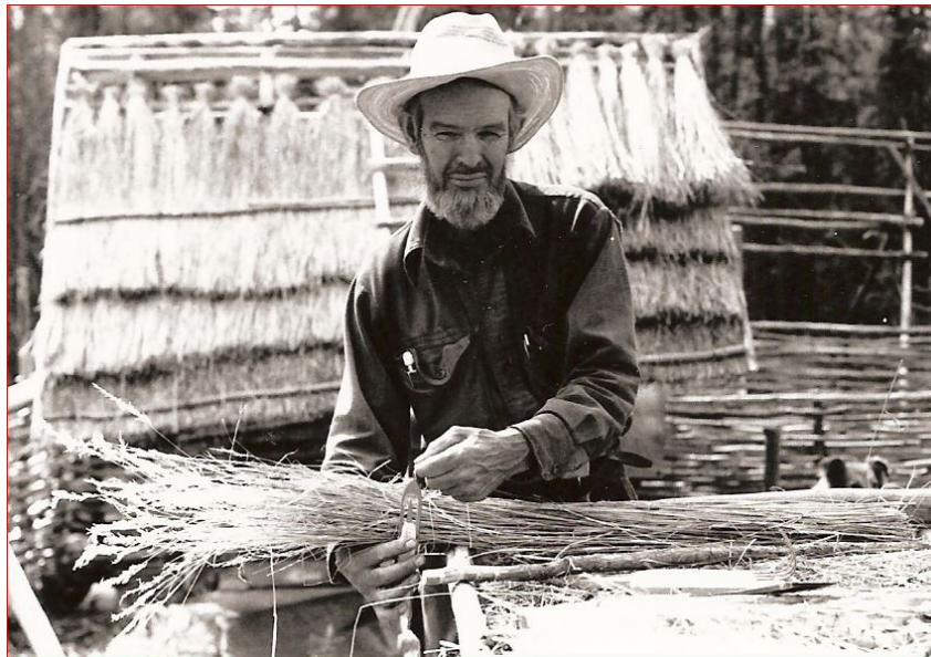
Oliver ties another bundle of thatch for the roof.
