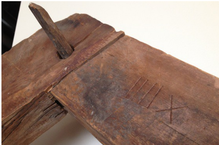
Mortise and tenon joint, pinned together with trunnel. Image:
