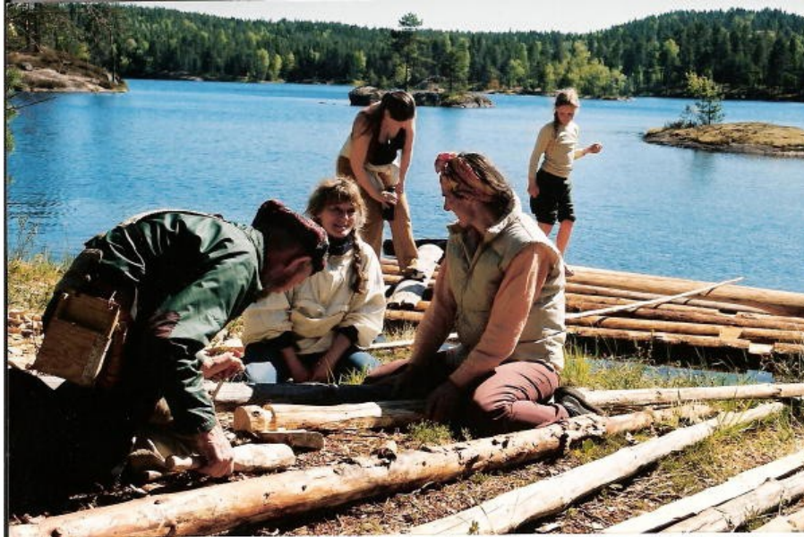
Heidi Dammann visits with a visitor as Oliver works with a chisel and a homemade club on a crosspiece. Note the channels in the logs that are floating in the lake.
