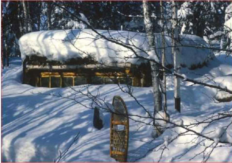
Ole Wik's first iglu, 1965. It measured 9' x 11' at the top frame. The flat roof was insulated with two layers of moss, separated by a sheet of Visqueen (as described above). Windows consisted of two sheets of Mylar inside and outside of a frame made of sticks. Entry was via a tunnel (opening shown in lower left corner. Image: Ole Wik
