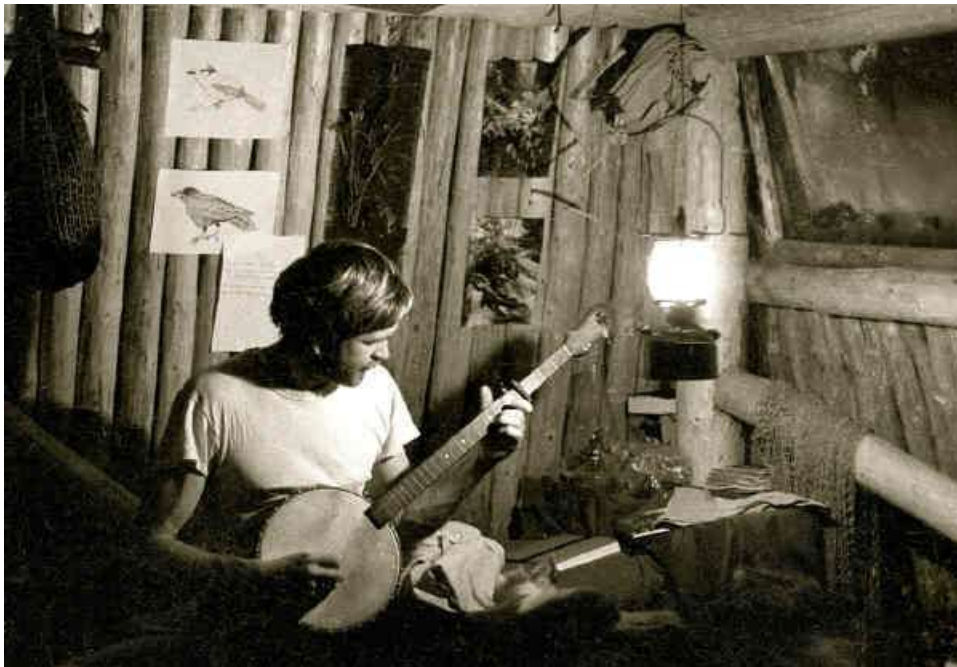
Ole inside the iglu described in the text, ca. 1970. The windows consist of one sheet of transparent vinyl. Note separate removable shutters made of Visqueen wrapped around both sides of simple pole frames. Image: Sasha Wik
