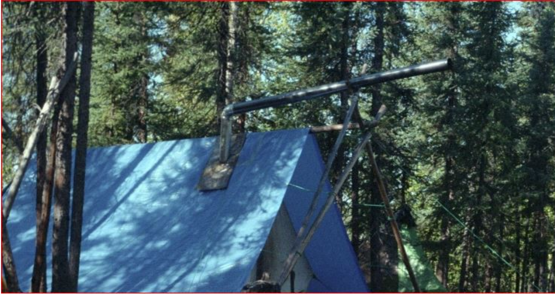
Visitor tent setup showing main shear pole, extended ridge pole, fly, stove safety, and second shear pole for stovepipe support. Image: Devta KhalsaI
