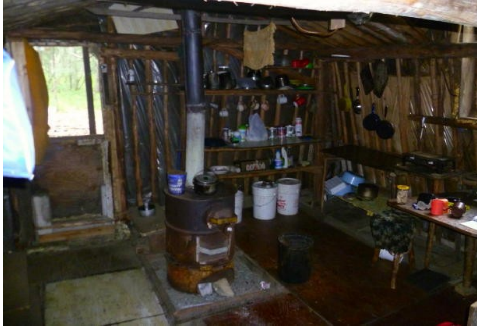
Interior, front area. Note the Visqueen vapor barrier.
