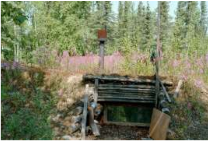
A window was set at ground level with dirt bermed up around it and over the top of the cabin, forming a thickly insulated mound.
