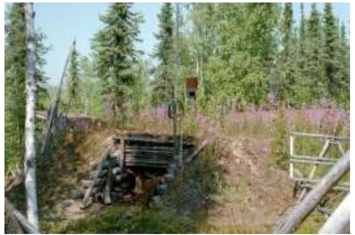
A window was set at ground level with dirt bermed up around it and over the top of the cabin, forming a thickly insulated mound.
