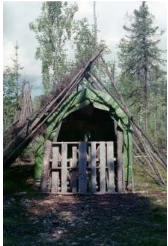
Spruce poles lean against the exterior shed walls with dry branches still on them serving as a bear deterrent.
